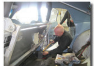
Setina's Todd Ginter installing the protective screen.
